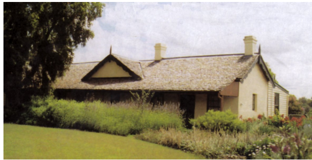
The 'Camden Cottage' (1820) (Belgenny Farm).
