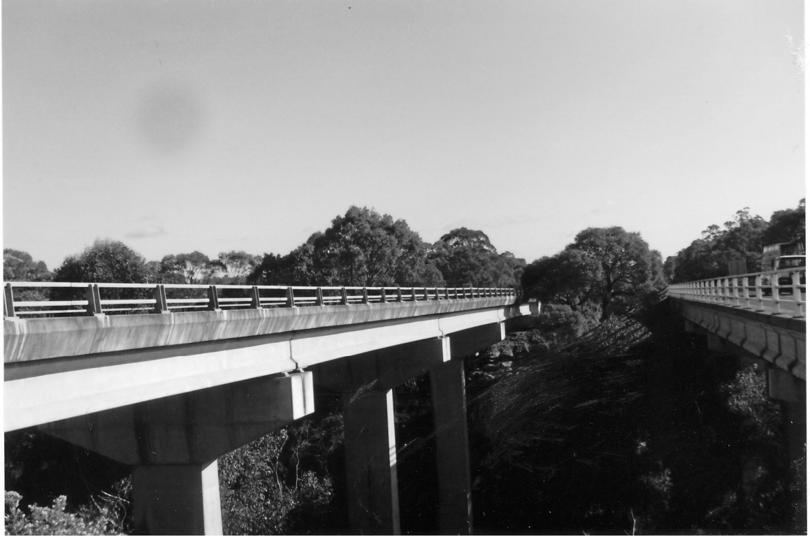
Present day double bridge replacement over Black Bob's Creek, 12 kms south of Berrima on the Old Hume Highway.
